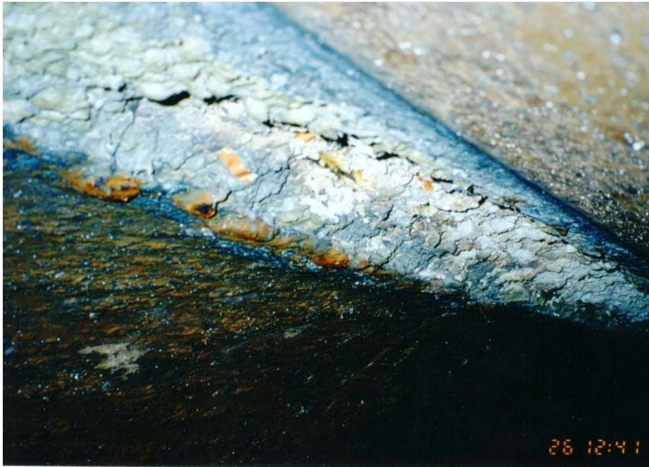
Figure 2-11. Crown Corrosion
