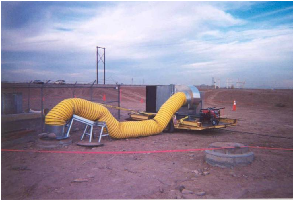
Figure 6-2. Air Extraction Skid for Sewer Ventilation Testing (Phoenix, Arizona)
