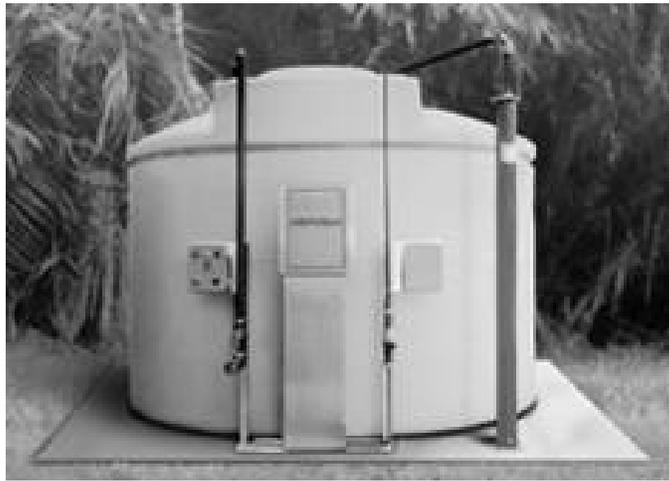
Figure 7-8. Bioxide Storage and Delivery System
